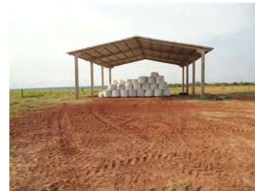
Hangar com adubo
